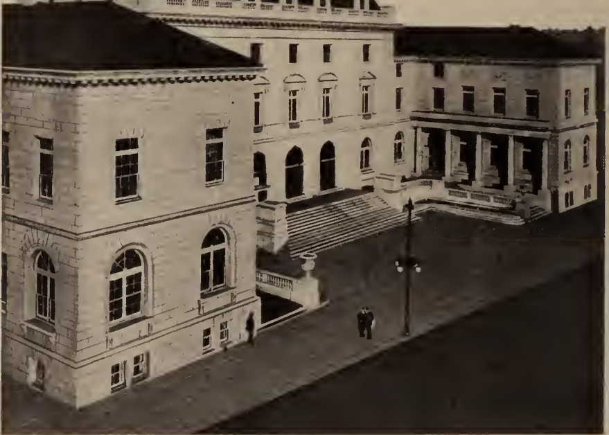
NEW CITY HALL, PORTLAND
